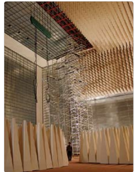
Rail system for the installation of pyramid absorbers
